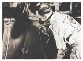
They thoroughly wash each new Fisher Body with an acid solution to remove all the dust and grease. Then, in a special booth, they spray on the "priming coat." After baking in an oven, the body moves on to another booth for a "glaze" coat—which is also baked on.
