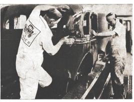
2 Under powerful floodlights in another booth, they then carefully inspect the "glaze" coat—and smooth it down with wet sandpaper. Where it's too thin—and at points where wear is heaviest—they "spot" glaze the surface.
